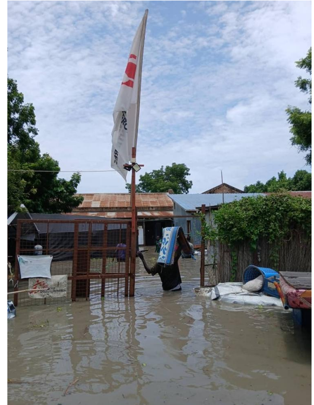
A flooded entrance to the MSF hospital in South Sudan
